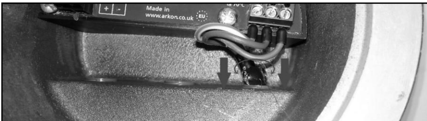
Pic. 3 Manipulation with the cable to achieve sufficient fill up of a cable gland
